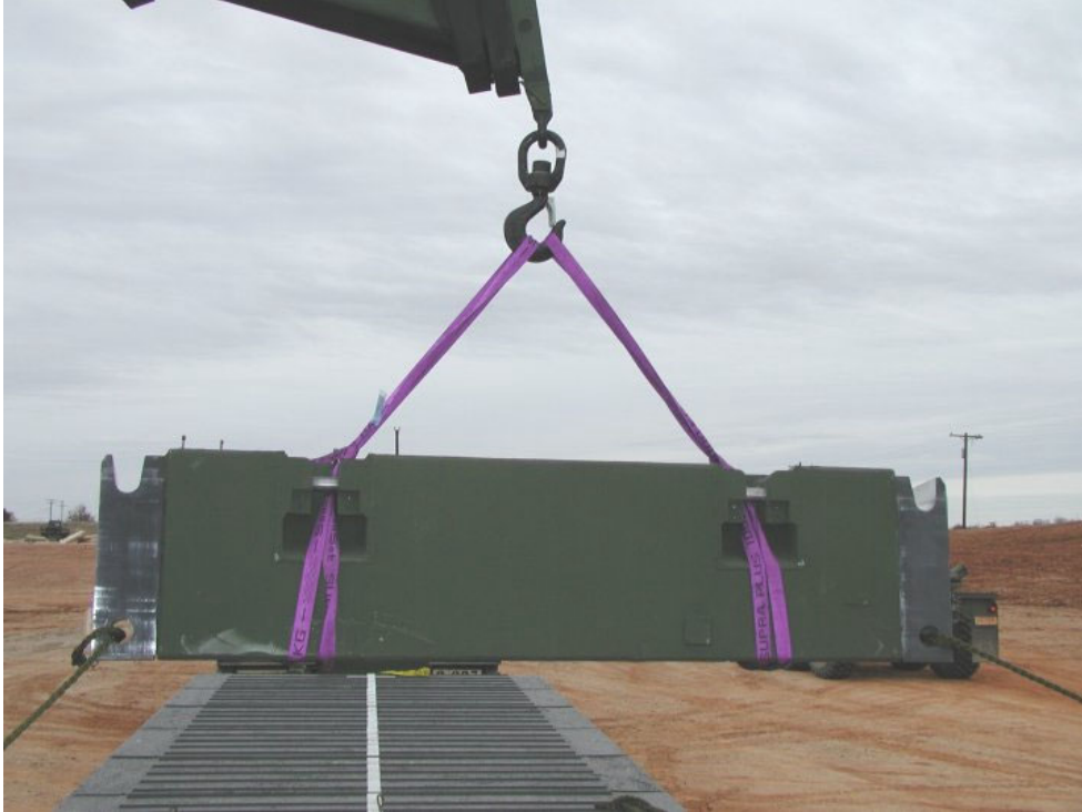
End Beam Slings Positioned
