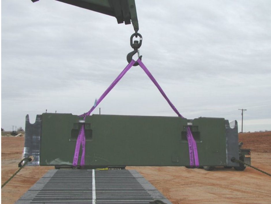
Figure 5. 3 Method for Slinging End Beam
