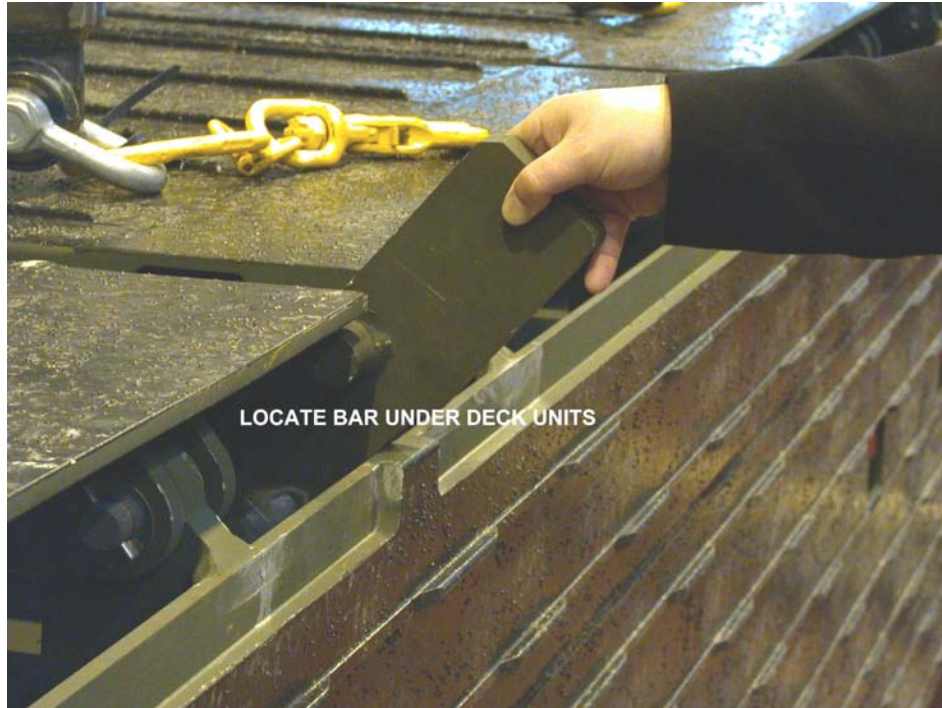
Figure 3. 52 Transport Aid inserted Under Deck Unit
