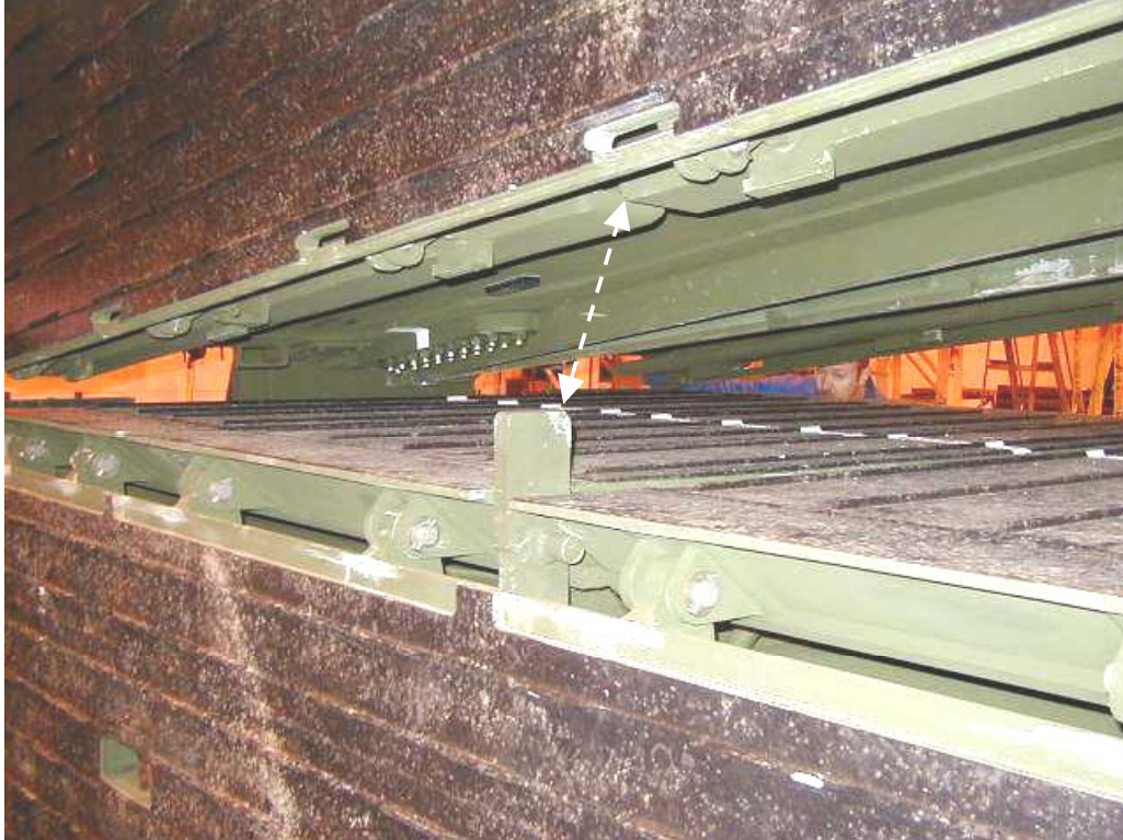
Figure 11. 102 Lower Top Module Onto Aid
