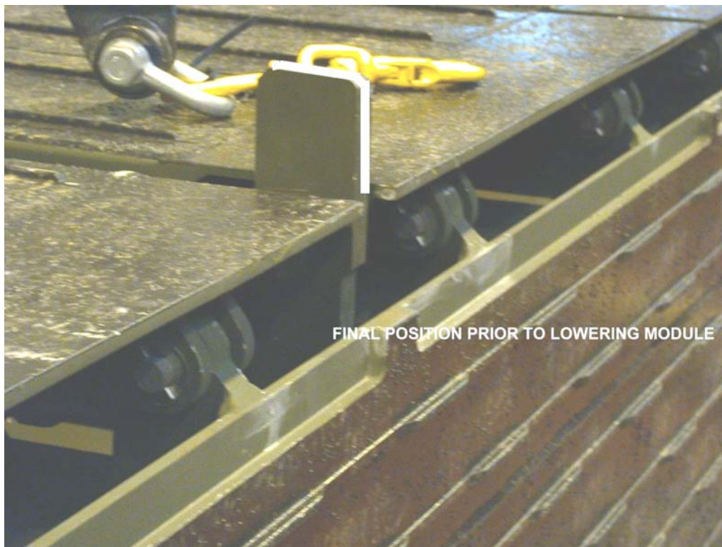
Figure 11. 100 Transport Aid Inserted Under Deck Unit
